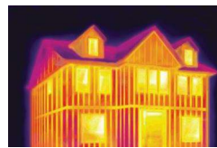
Before Cavity insulation only
