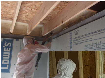
Air sealing & insulation for floor perimeter
