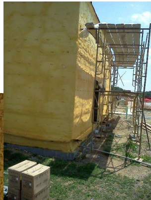
Ci/WRB/AB on school (masonry cavity wall)
