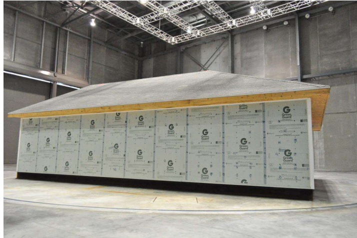
Foam sheathing and taped WRB joints survived exposure to hurricane force winds with no damage (even with siding removed)
