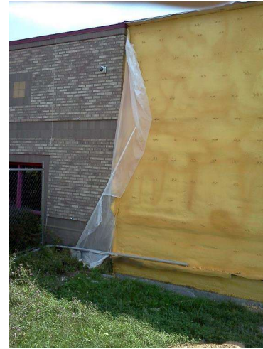
School Addition – Masonry/SPF/Brick cavity wall
